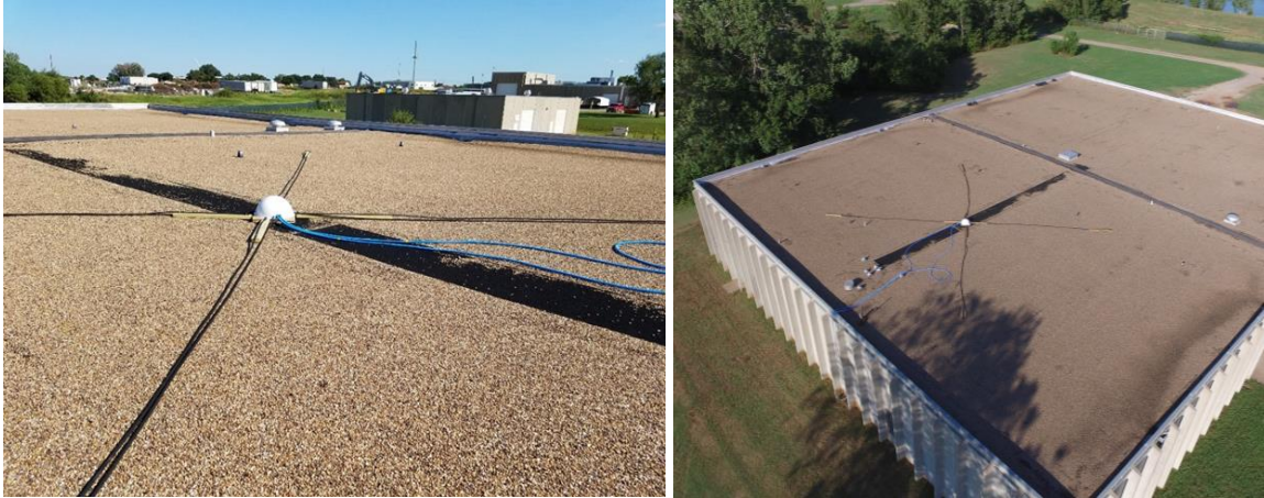
Figure 17: (left) Final configuration for the roof top microphone deployment with soaker hoses spread out in an 'X' shape. (right) Aerial view of the roof top deployment.
